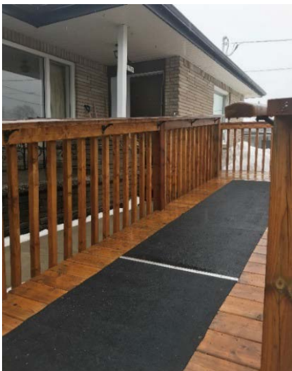
Figure 3.6 Ramp into Haley House
